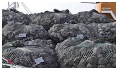
Submerged breakwater construction material (Filling material: Steel slag hydrated matrix)
